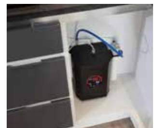
Under counter heating tank
